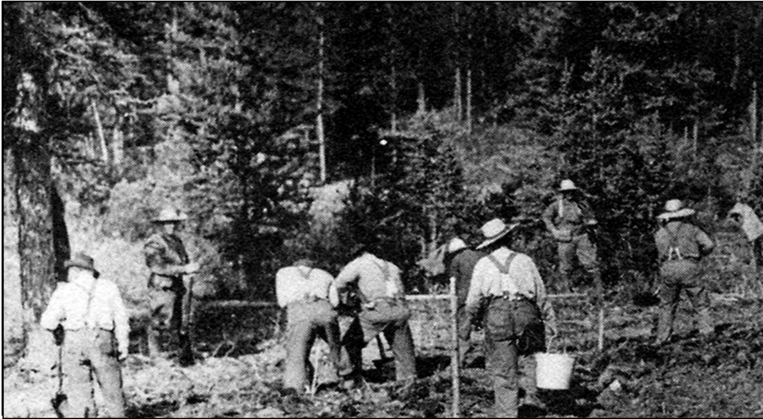
Construction of motor road from Banff to Lake Louise, circa 1915
